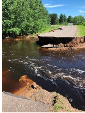
Pease Road at James Road Monday, June 18th
