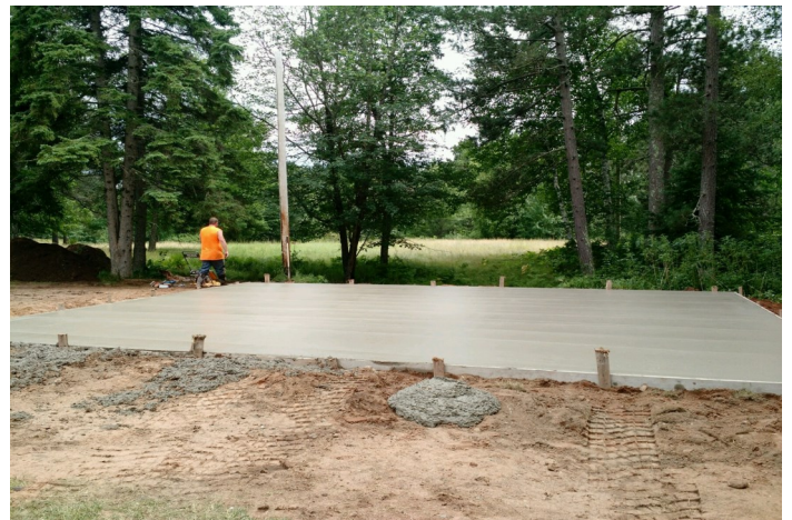
The slab is poured for the Pease School
